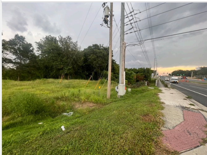
9. Pole-mounted transformer
